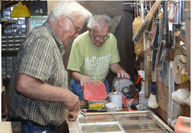
At right the Klauer brothers are replacing the glazing putty on one of the windows that we are restoring.
