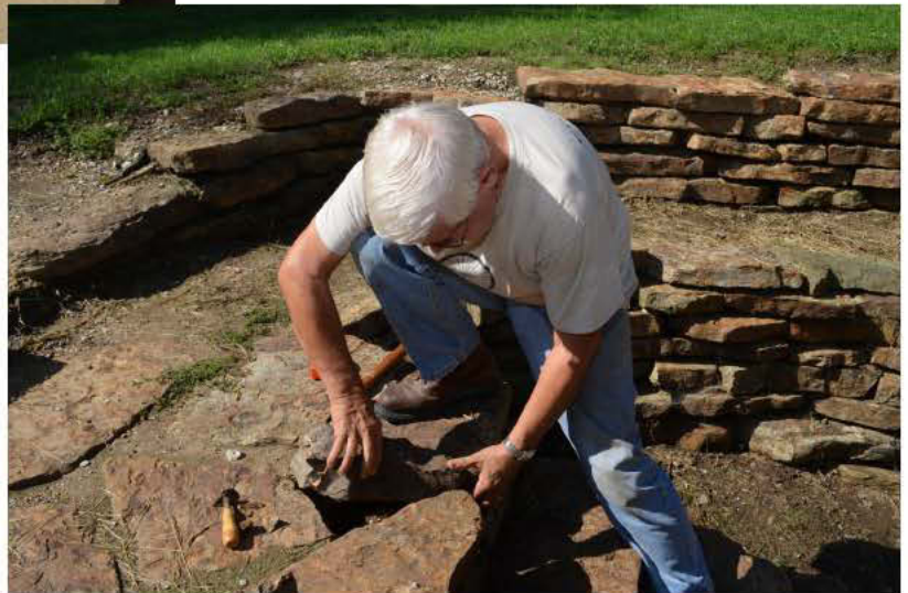
Dick Stoltenburg is our stone mason. Here he is doing the final fitting of a replacement stone on the boiler room steps.
