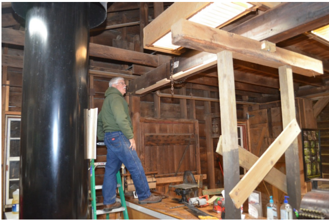
At this point the steel plate is almost in place. It is held against the wood beam by wood clips. Note the safety chains that prevent it from falling.
