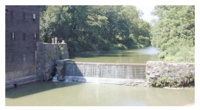
The current dam was built in the 1960's. The original dam was a timber and rock rubble structure about 5' higher then the current one. One of the Friends of the Mill future projects will be to raise the level of the dam. As it now stands there is not enough head to power the turbine properly.
