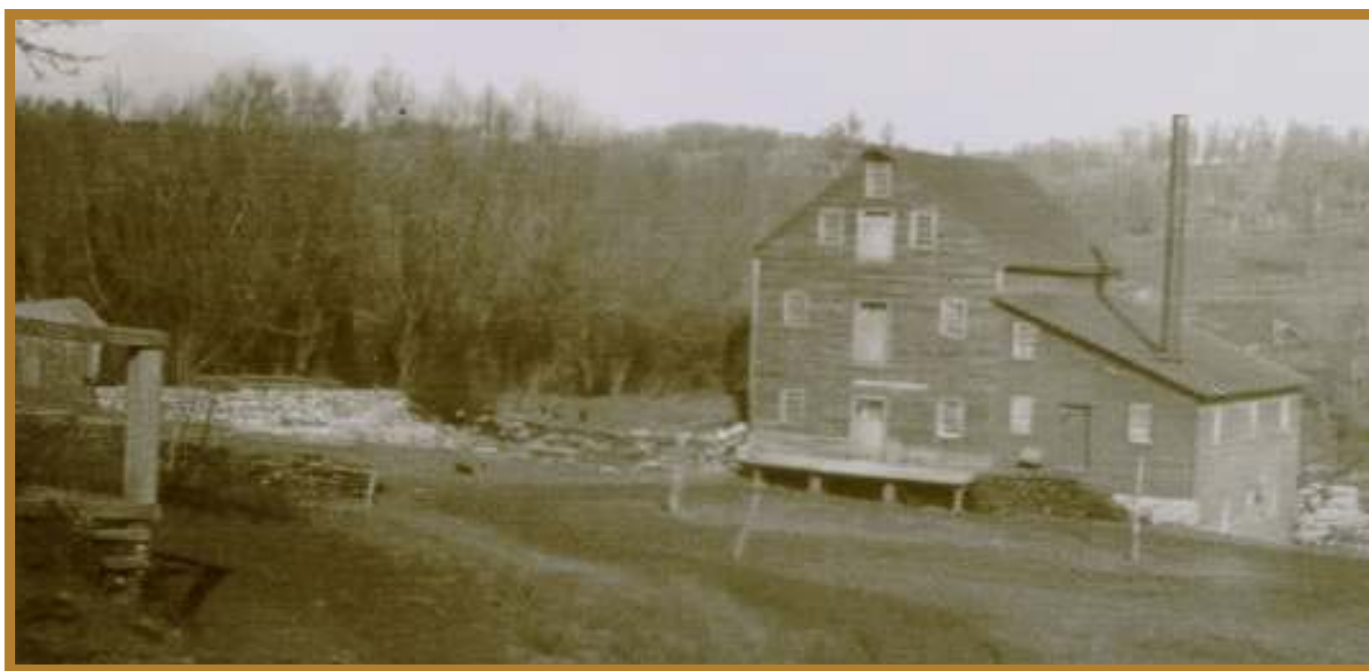
Pine Creek Grist Mill prior to WW1. Note the wagon loading dock and the stack of fire wood for the boiler.
