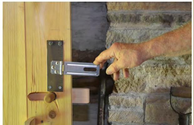
Clarence Klauer and Don Stoltenburg repaired the broken cabin door. The steel plate they installed to reinforce the hasp is shown above.
