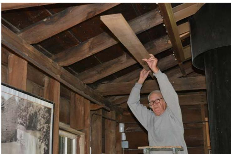
John Bixby is installing a board that will hold the new LED fixture in the rear of the country store area. Two of us do the preparation work for the fixtures while the electricians follow behind to do the installation.
