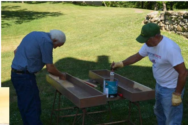
Dick Stoltenburg is cleaning the 48" pulley that drives the corn mill to prepare it for being treated with wood preservative.
