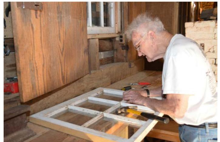
Dick Klauer is repairing the basement window that vandals had broken. He had to fabricate a new mullion for the window.
