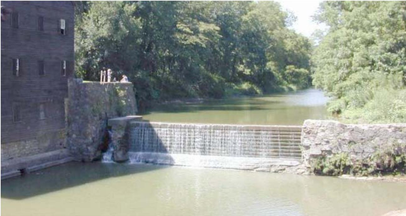
The current dam was built in the 1960's. The original dam was a timber and rock rubble structure about 5' higher than the current one. One of the Friends of the Mill future projects will be to raise the level of the dam. As it now stands there is not enough head to power the turbine properly.
