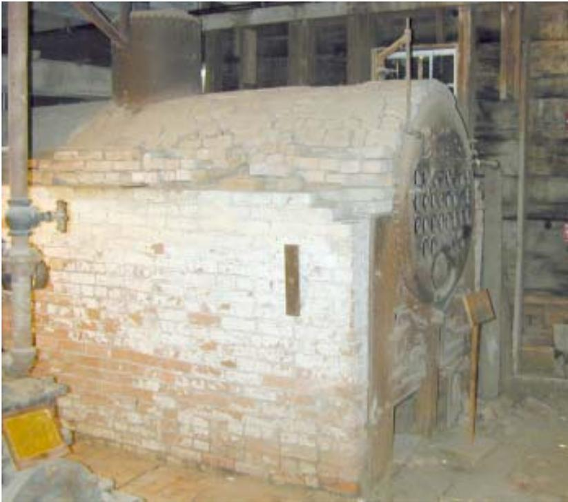
Some time in the late 1870's a steam engine and boiler were added to power Pine Mill. It powered the mill during times of low water in the creek and handled the additional load of the new roller flour mill.
